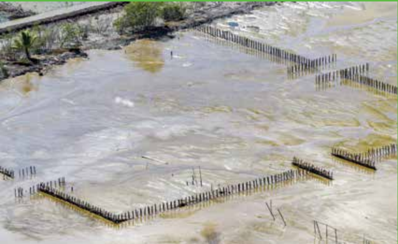
Sediment Trapping Units installed along the coast of Suriname promote sediment deposition and create conditions for halting and reversing erosion, including by creating a habitat for new mangrove juveniles.
